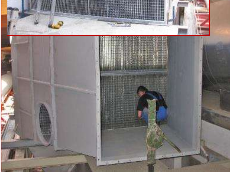
Air / air HX: 5 mm plate spacing
